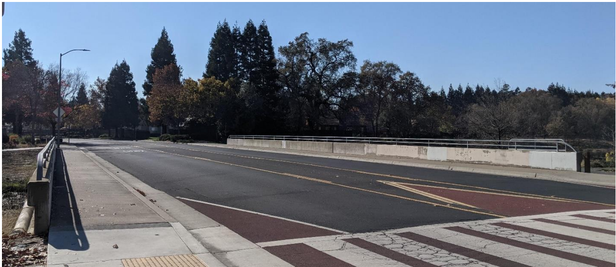
The east wall is approximately 151' in length
